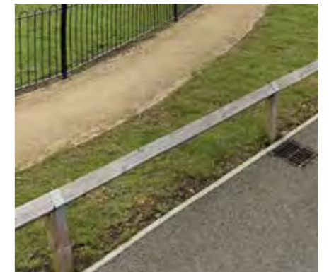
Timber Knee Rail Fence
